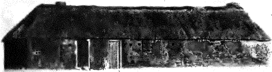
GUARD HOUSE, GRAHAMSTOWN
